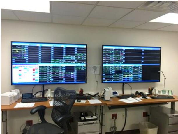
Figure 3: Poste central de monitoring cardiaque
